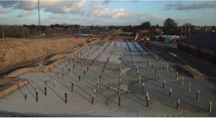
IT-DSP™ In-situ Full-scale IT-DSP™ project Teckomatorp, Sweden.
